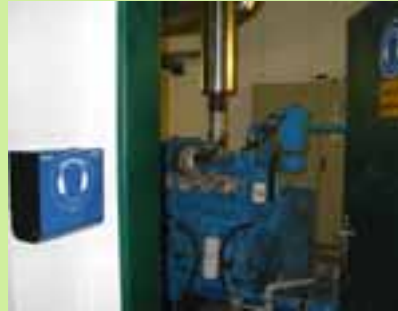
Notstromaggregat
